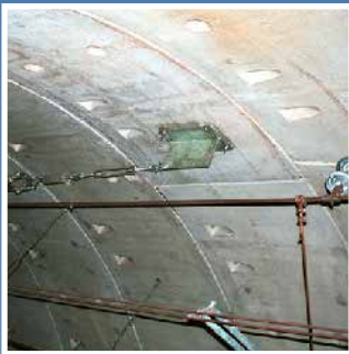
Sydney Airport Rail Link
